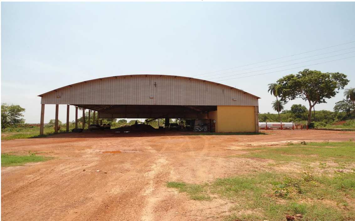
Tailings Material Recovery Plant Mineração Tuiuiu - Brazil – Frontier/Four Star Producing gold by pyrometalurgy
