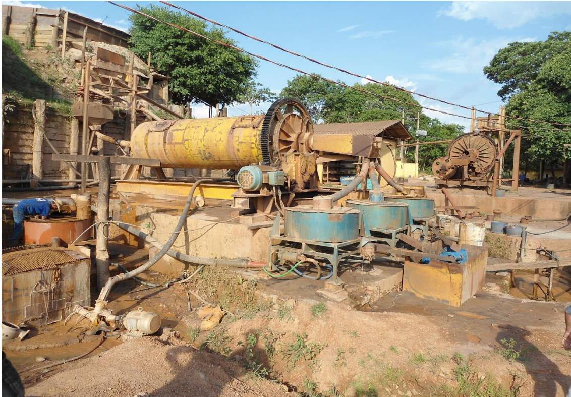
Mineração Tuiuiu - Brazil – Frontier/Four Star Producing gold by pyrometallurgy Existing Gold Mining Operation – seeing ball mills and gold centrifuges
