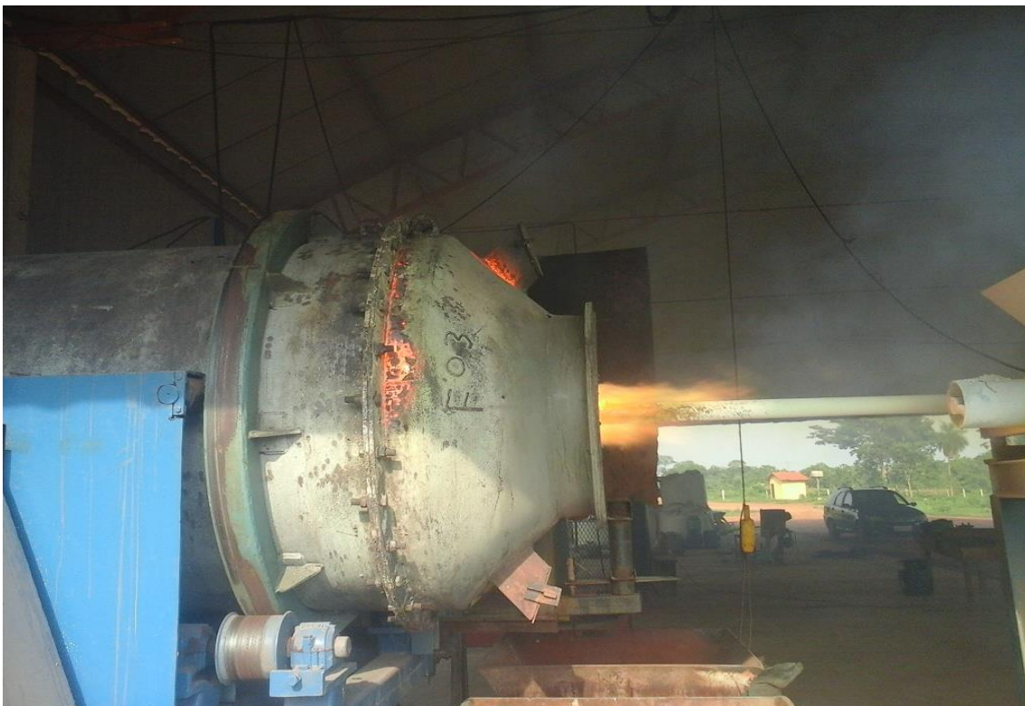
Mineração Tuiuiu - Brazil – Frontier/Four Star Producing gold by pyrometallurgy Poconé – MT – Refractory failure on smelter side
