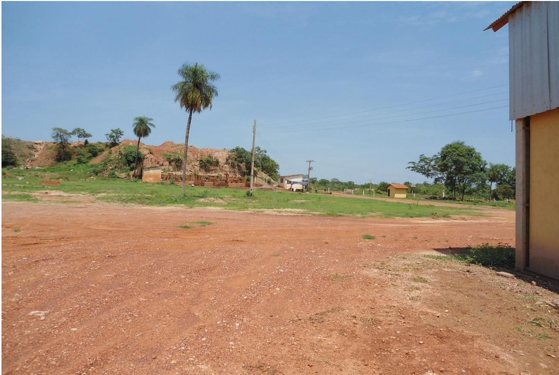
Mineração Tuiuiu - Brazil – Frontier/Four Star Producing gold by pyrometalurgy A new tailings concentration plant will be assembled here
