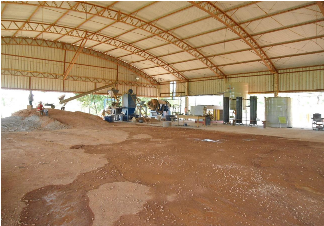
Mineração Tuiuiu - Brazil – Frontier/Four Star Producing gold by pyrometallurgy Our Concentration/Smelter Plant – General View
