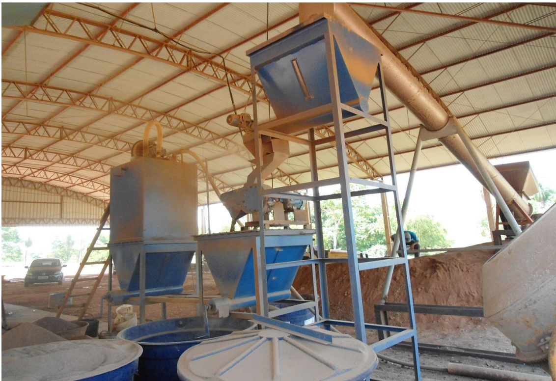
Mineração Tuiuiu - Brazil – Frontier/Four Star Producing gold by pyrometallurgy Frontier's/Four Star Concentration Plant
