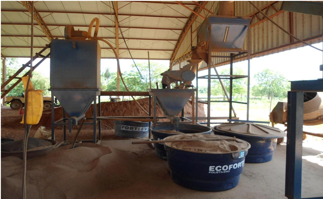
Mineração Tuiuiu - Brazil – Frontier/Four Star Producing gold by pyrometallurgy Dry Concentration Plant
