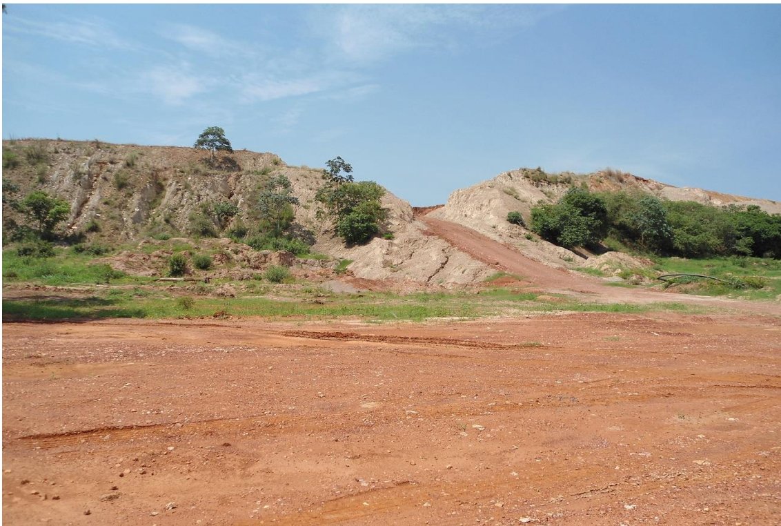
Mineração Tuiuiu - Brazil – Frontier/Four Star Producing gold by pyrometalurgy Tailings Dam
