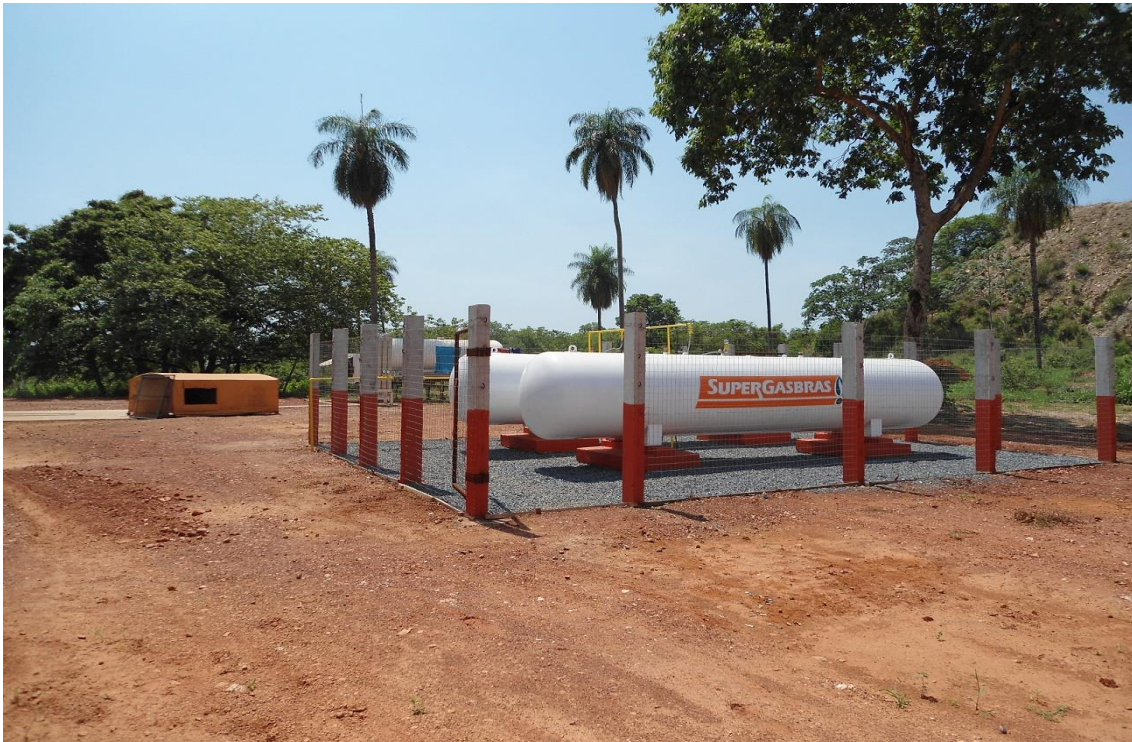
Mineração Tuiuiu - Brazil – Frontier/Four Star Producing gold by pyrometalurgy Fuel Tanks – Our fuel are GLP – Gas
