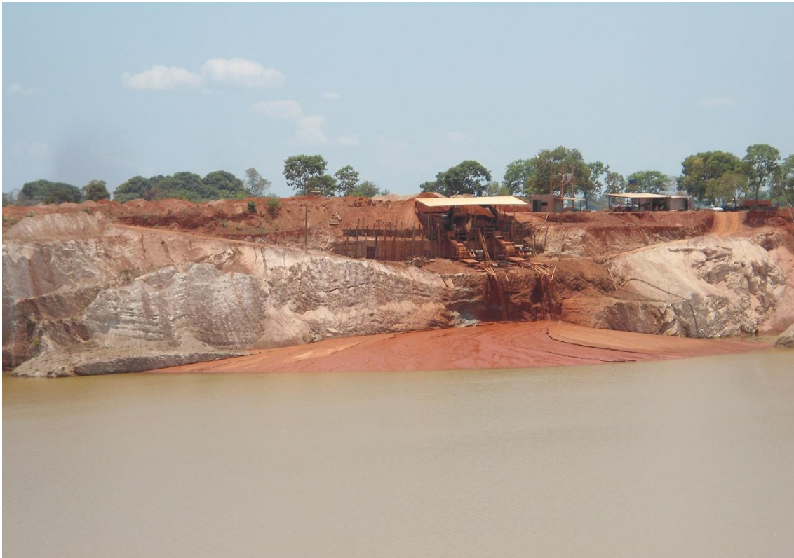
GOLD PLANT IN OPERATION
