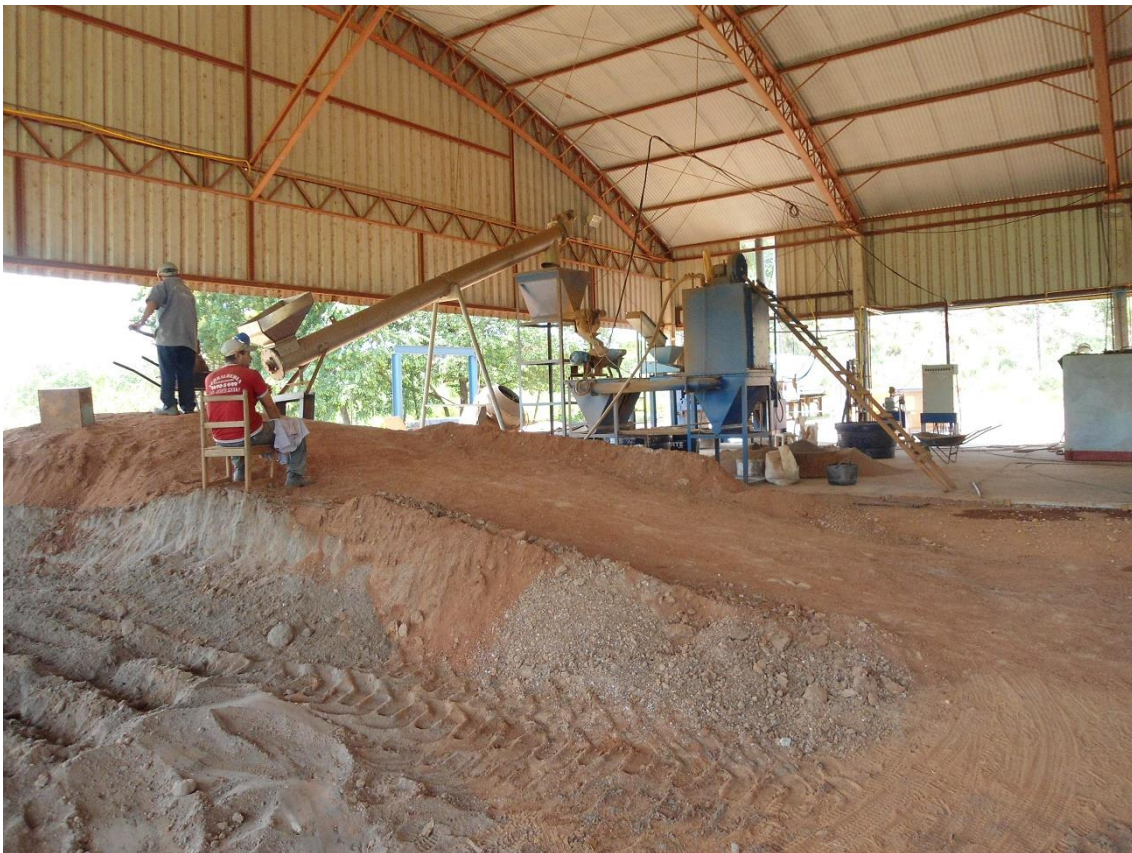
Mineração Tuiuiu - Brazil – Frontier/Four Star Producing gold by pyrometalurgy Frontier's Technology – Dry Concentrating Plant
