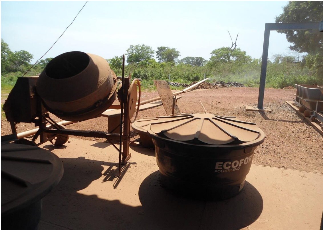
Mineração Tuiuiu - Brazil – Frontier/Four Star Producing gold by pyrometalurgy Waisting Pounder Dust showing on the White pipe overthere
