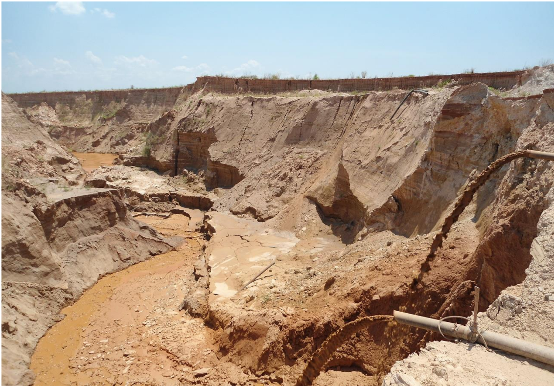
COUNTRY TAILINGS DAM TODAY
